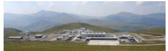
Compound for the Azeri-Turkish pipeline
